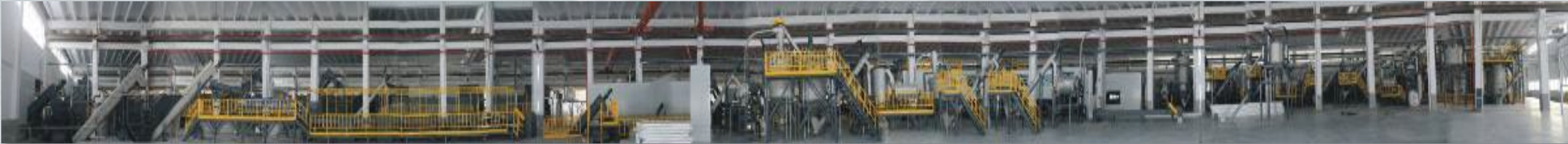
200 meters long of PET flakes processing line
